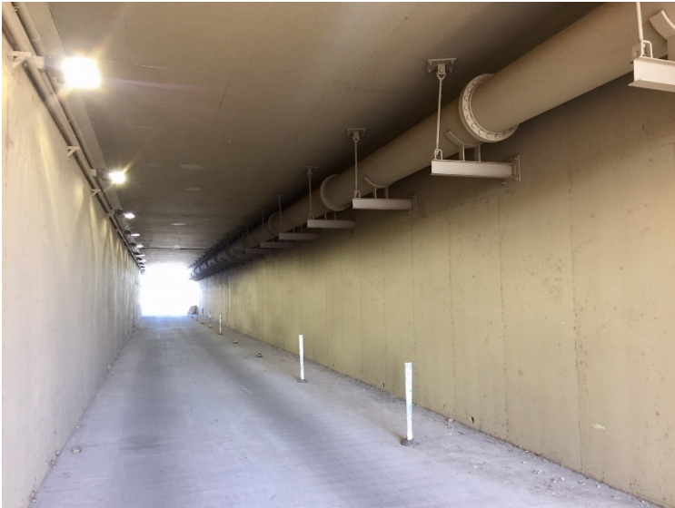
Interior of the underpass
